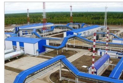
Oil Pump Station "Tayezhnaya", Transneft
