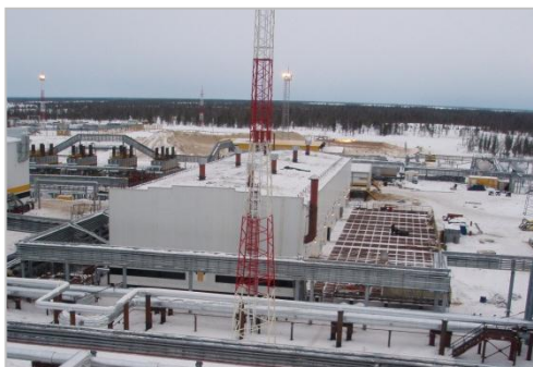
Oilfield Pump Station 2, Vankor oilfield, Rosneft
